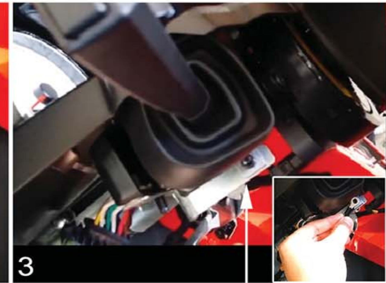
3 Locate the hex key GROUND bolt under the steering column. Attach the Keyless Ignition Ground lug to the bolt and tighten.
